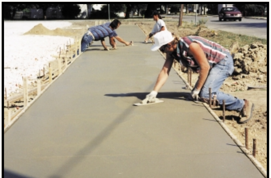
Workmen finishing concrete is a common sight around campus.
