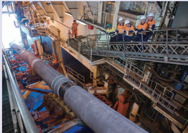
Start of construction of gas trunk pipeline for Ichthys LNG Project
