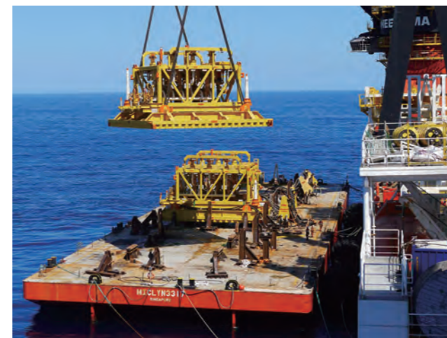
Subsea wellhead assembly installation operations
