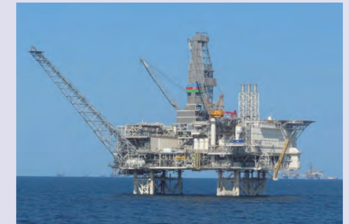
Production platform for the Chirag Oil Project in the ACG oil fields concession in the Caspian Sea
