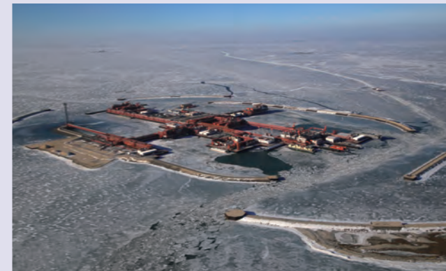
Production facilities at the Kashagan Oil Field
