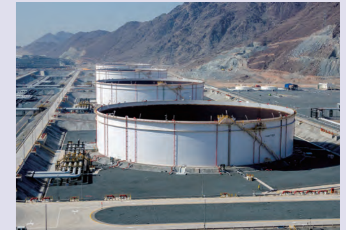
Fujairah Terminal used to ship production (Murban oil) from ADCO Onshore Concession
