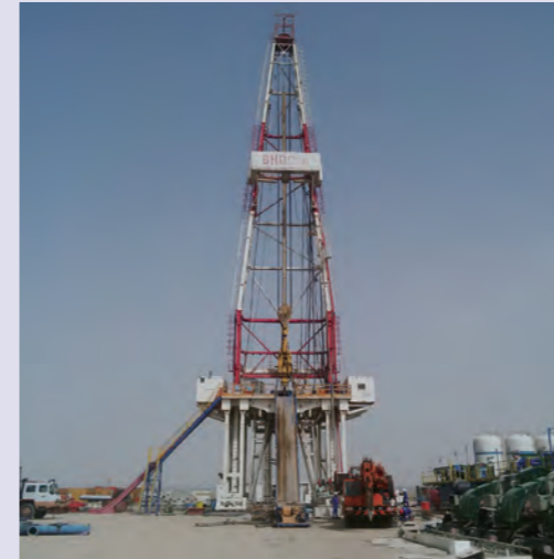
Drilling wildcat wells at Exploration Block 10 in Iraq
