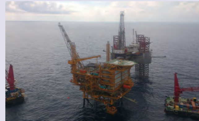
Oil production started in the offshore production facilities at the Ruby Gas Field, Indonesia
