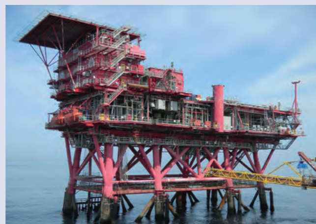
Decommissioning work of platform at the Offshore Iwaki Gas Field
