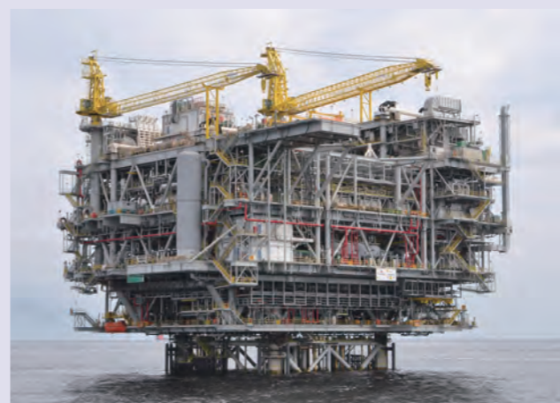
Production facilities at the Offshore Angola Block 14
