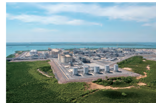
Panoramic view of onshore LNG plant
