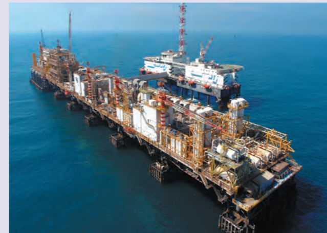
Production facilities at the Upper Zakum Oil Field
