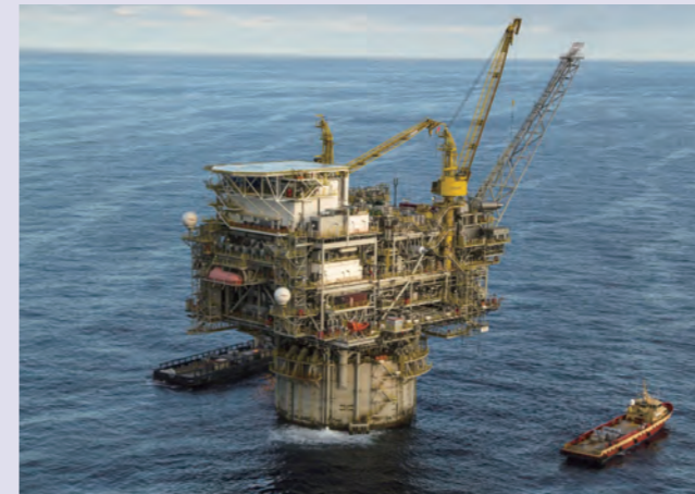
Production facilities at the Lucius Oil Field
