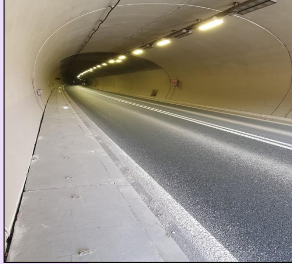
Figure 3. Tunnel pipe for motor vehicle traffic
