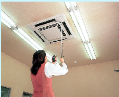
Check airflow rate of air conditioner
