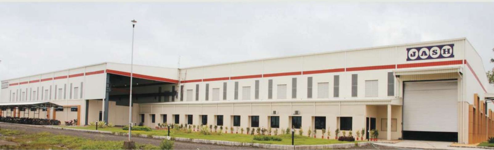
Jash Engineering Ltd, Pithampur
