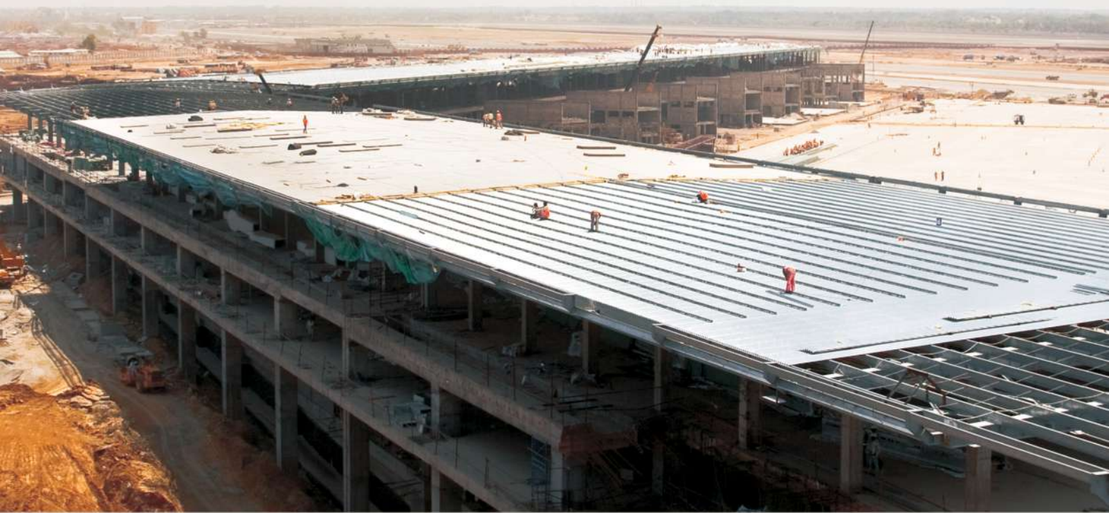
Standing Seam Roofing System - IGI Airport Terminal 3, PIERS
