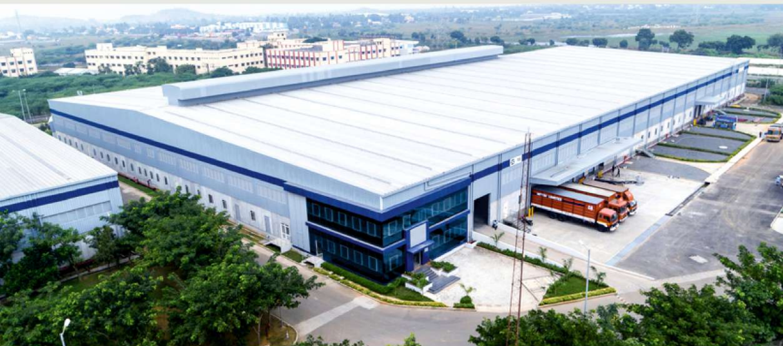
IndoSpace, Logistic Parks at Multiple Locations
