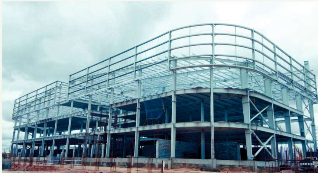
Typical Primary and Secondary Framing Systems
