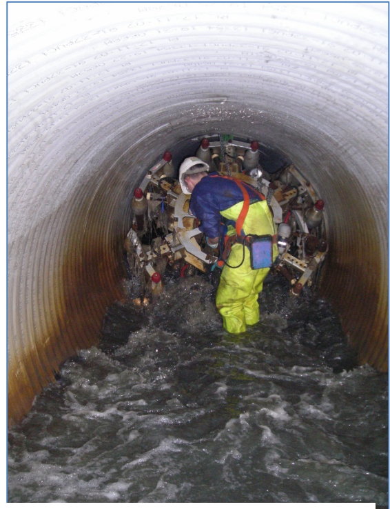
Interflow employee working with Rotaloc pipeline in live flow.
