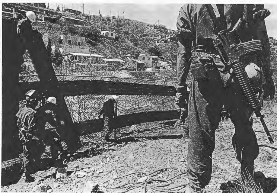
The military constructs a wall separating Nogales, Ariz. from Mexico.
