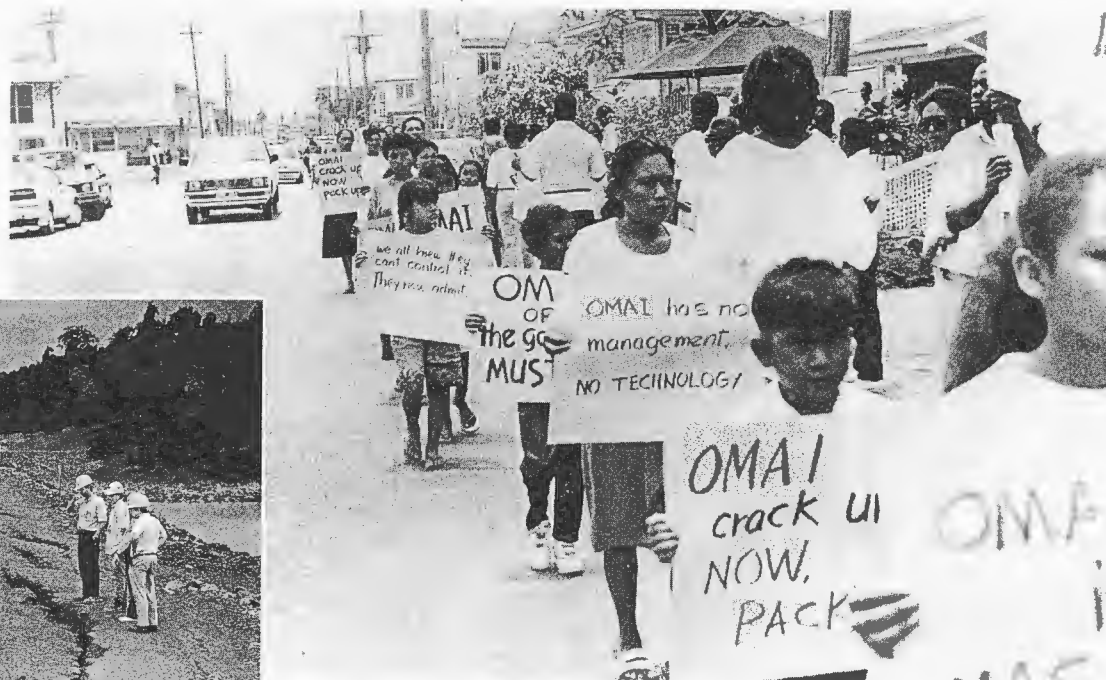
August 1995. Cracks in the tailings pond wall (II). Protesters at Omai's Georgetown offices (top).
