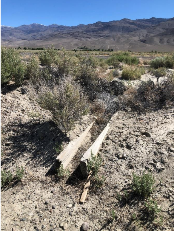
Wooden box culvert along the Carson and Colorado Railroad grade
