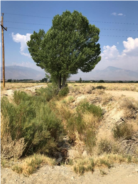
Carson and Colorado Railroad grade, looking downstream from McNally Return Ditch crossing
