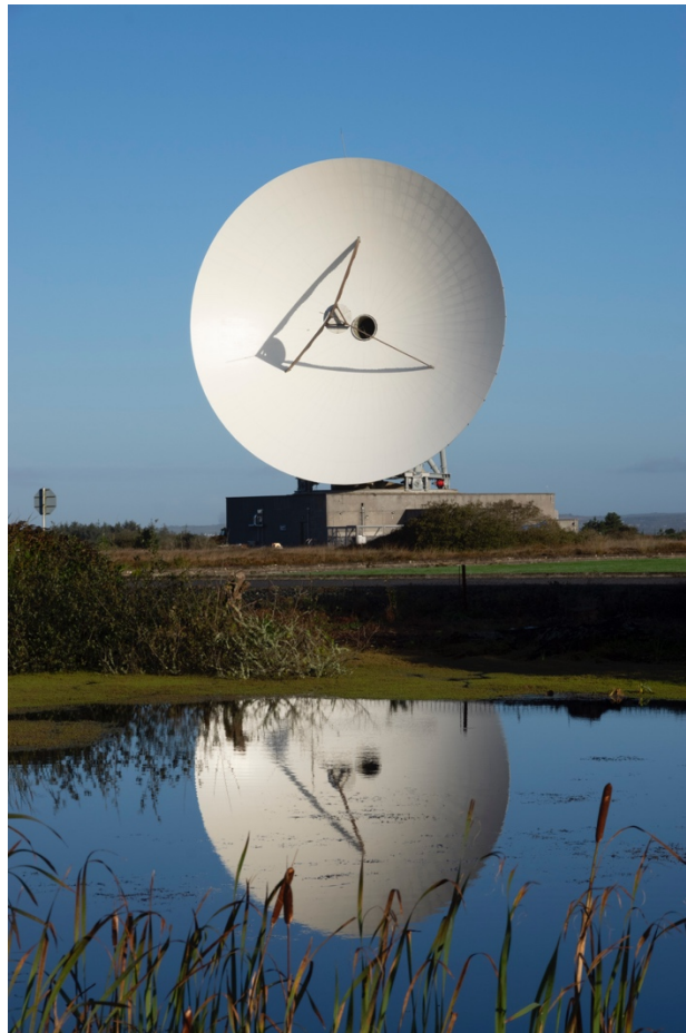
Figure 3.8-2. Goonhilly's GHY-6 32m S- & X-band antenna. Picture Credit: Goonhilly Earth Station Ltd
