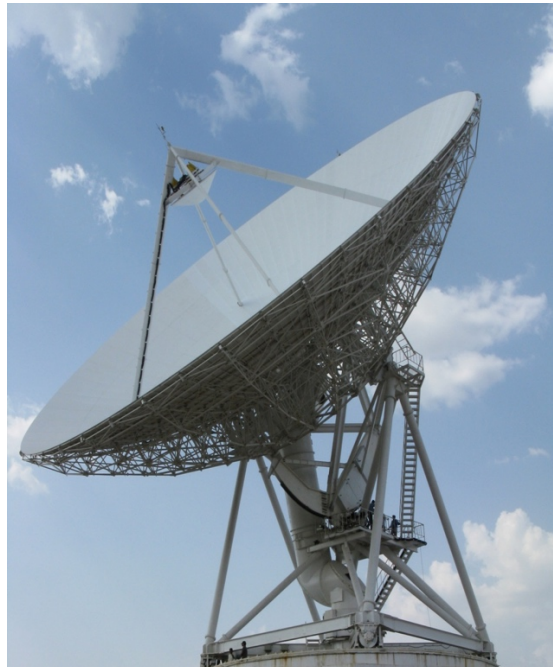
Figure 3.3-7. The IDSN-32m antenna
