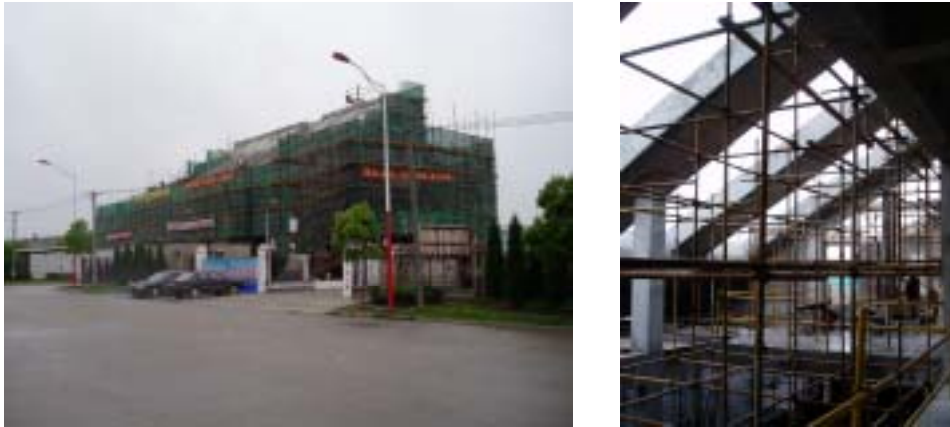
Figure 2.5 Site photos showing the current progress of the SRIBS Eco-Building
