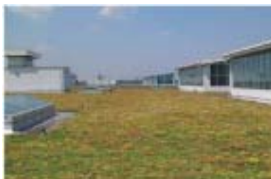
Fig 5: Building specific strategies, like green roofs, can help optimize storm water infrastructure. (Rouge River Ford Plant, WMD+P).
