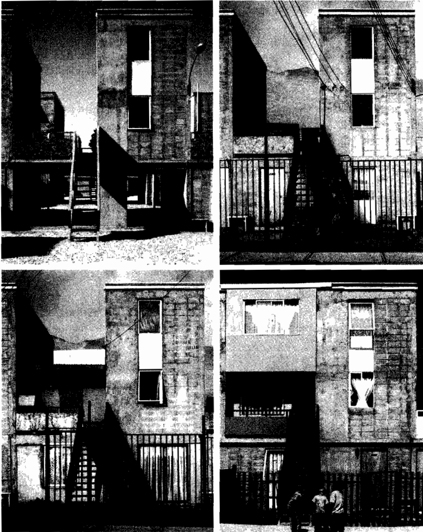
Figure 10: affordable housing in Iquique, Chile, by Elemental, an example of a house expanded by local resident.
