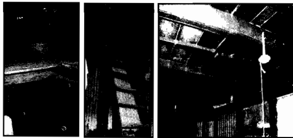
Figure 3: Temperature and humidity data logger position in upper space (right); Entry from indoor space to upper space (left); Wooden ladder for entering to the upper space (middle).
