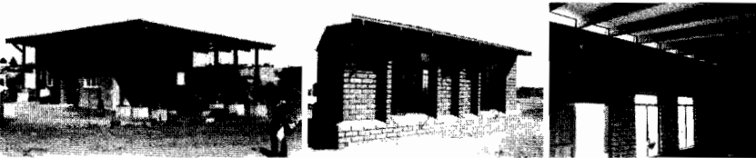
Figure 5: Three projects by the UEC: (a) and (b) day care centers in Bloemfontein and (c) a tourism craft center in Gariep Dam.
