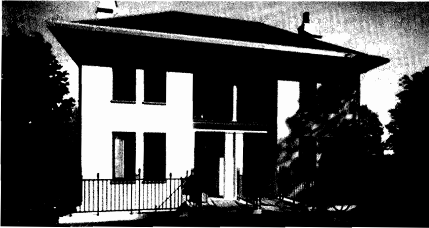
Figure 6. Prince's Foundation Eco House.
