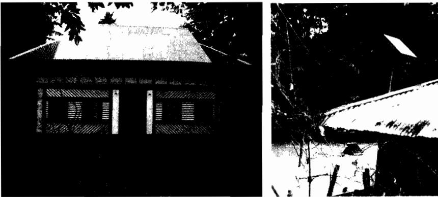
Figure 6: Bangladesh traditional house and Solar panel over its roof.
