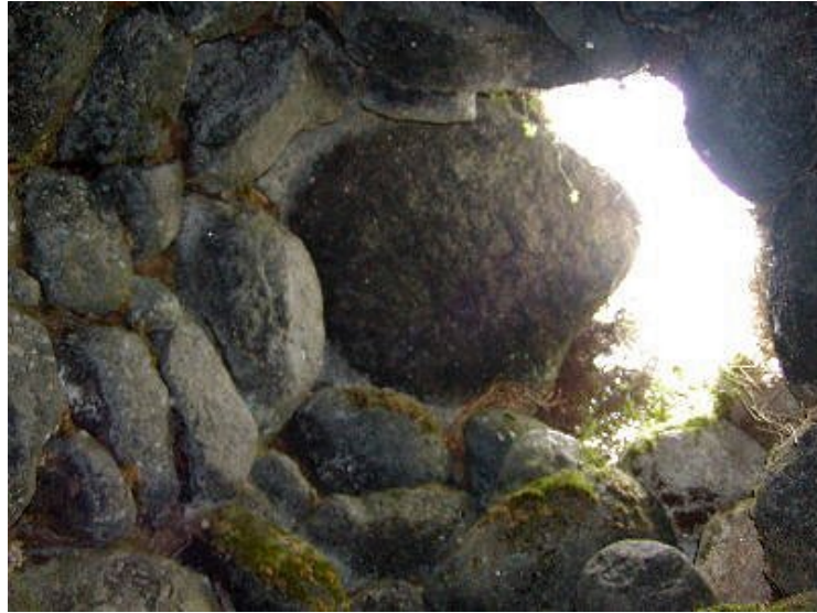
A hole in the corbelled roof photographed from inside the sweathouse at Annacarney in county Wicklow, far from the main distribution, but in a remote location. (Click the picture for more.)
