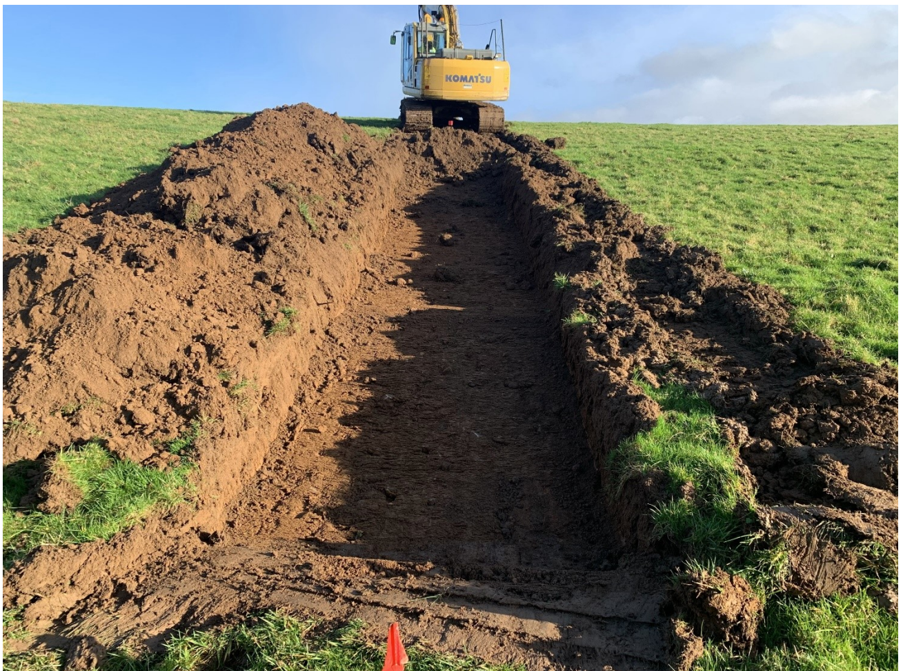
Plate 12: Test Trench 10, facing south-east
