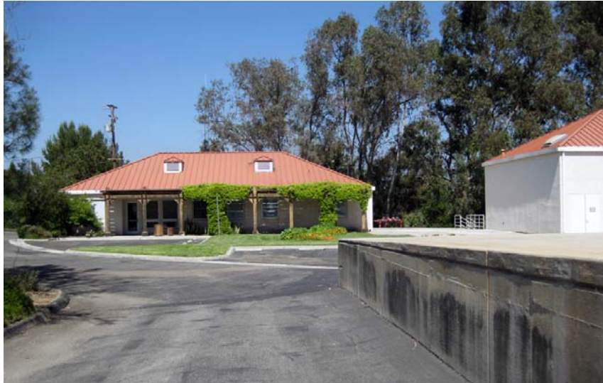
(a) Existing office, storage building, and partially-buried 3.4 MG reservoir, looking northeast.
