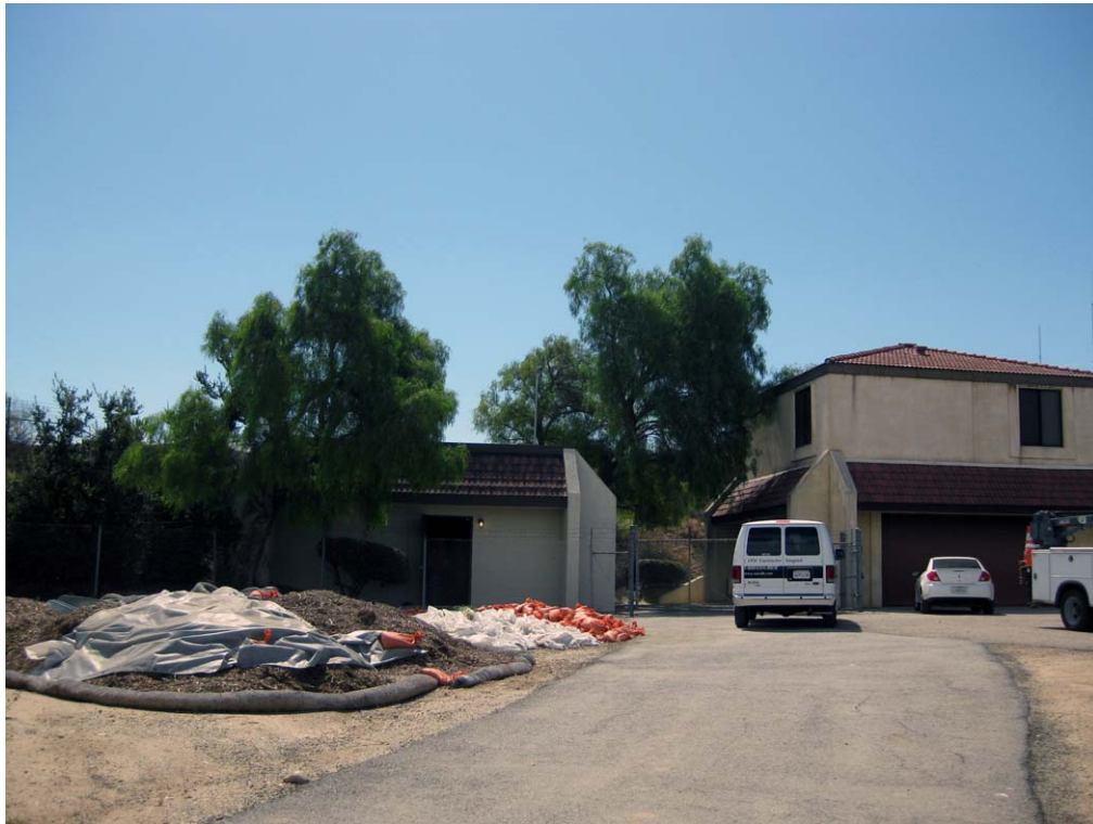
(a) Existing Baker/Irvine Lake Pipeline Intertie Facility (on left), looking east.
