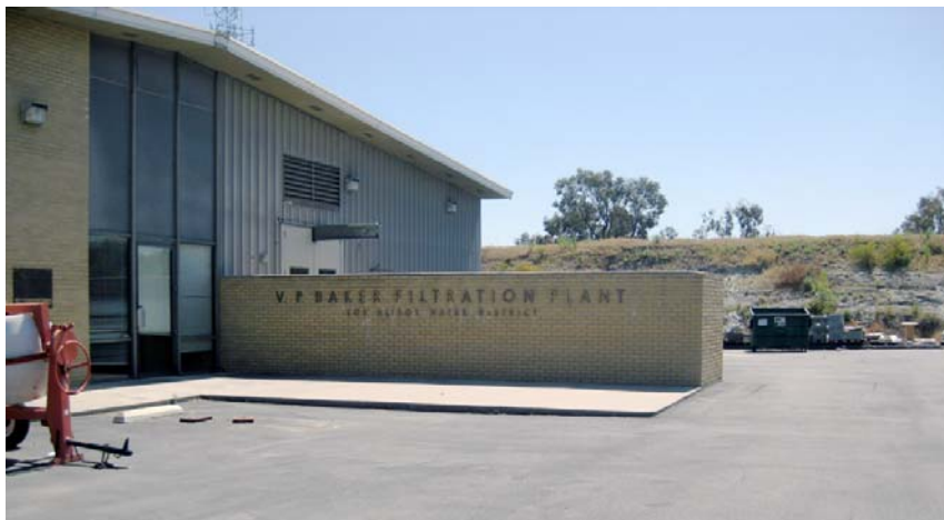
(c) Existing filter building, looking southwest.
