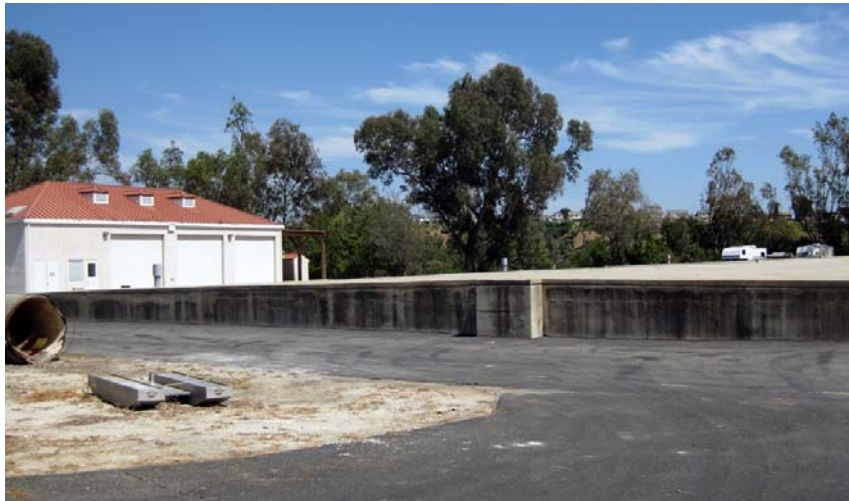
(b) Existing storage building and partially-buried 3.4 MG reservoir, looking southeast.
