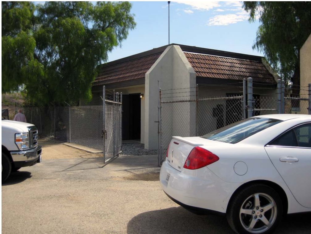
(b) Existing Baker/Irvine Lake Pipeline Intertie Facility, looking northeast.
