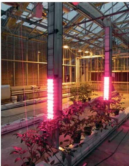
Figure 10. The young tomato plants in the foreground are receiving supplemental side lighting from LED towers during the cloudy days of January in Indiana. Only the lowest LED panel is energized while the plants are small to save electrical energy. Unlighted control and HPS-supplemented plants are being grown for comparison in the background.
