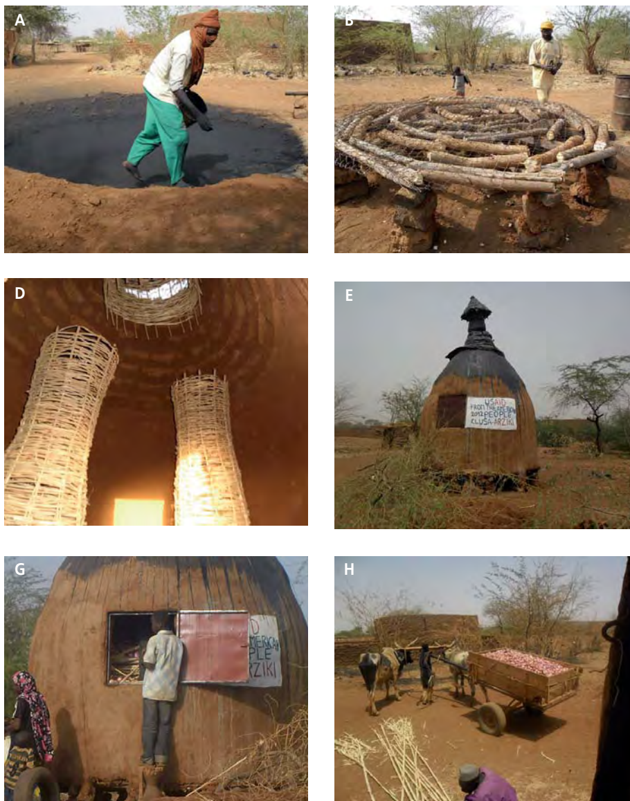
Figure 5. A. Spreading charcoal and salt to repel termites. B. Constructing the base covered with wire net on top of supporting stones. C. Constructing the store and plastering with mud. D. Inserting two aeration chimneys. E. Store is ready. Note chimney and tar-painted top. F. Loading the store: one layer of onion bulbs and one layer of millet straw. G. Periodical inspection for spoiled and sprouting onions. H. Six months later. Taking onions to market...
