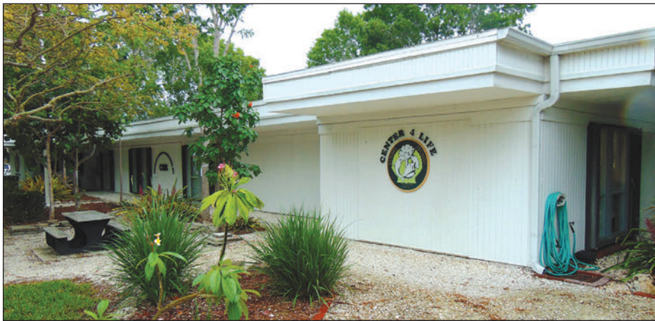
The existing Center 4 Life/Senior Center facility on Library Way photo by Jeff Lysiak
