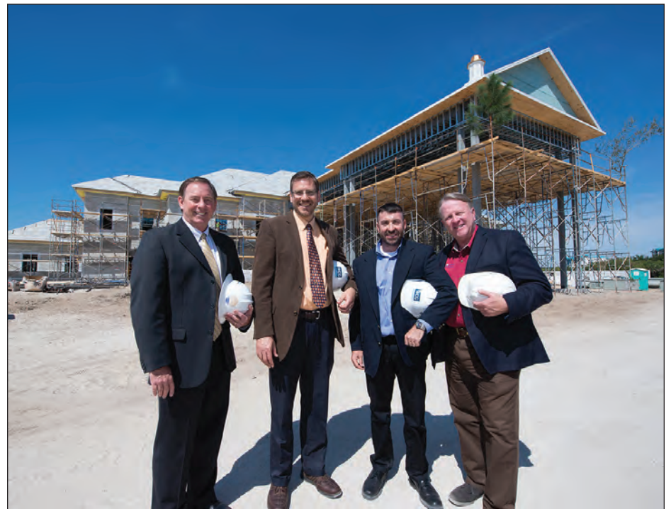
From left, Scott Moore, Shell Point chief operating officer; Fred Edman, president, Wright Construction Group; Scott Loiacano, project manager, Wright Construction Group; and Bob Southern, Shell Point director of project, at The Shell Point Clubhouse topping-off celebration photo Rich Cerrina/Shell Point Retirement Community
