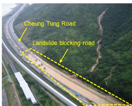
Figure 64. Debris flow obstructing Cheung Tung Road on Lantau Island, Hong Kong
