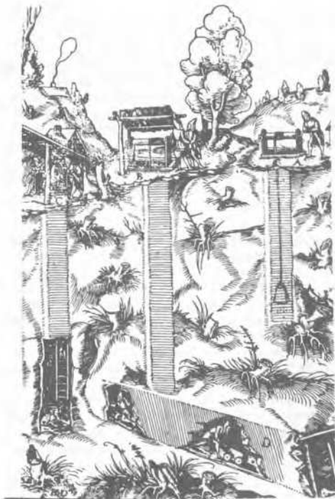
Fig. 111 - Techniques involved in the excavation of a mine, after Agricola (1556). Note the winches and the trolleys with four wheels.
