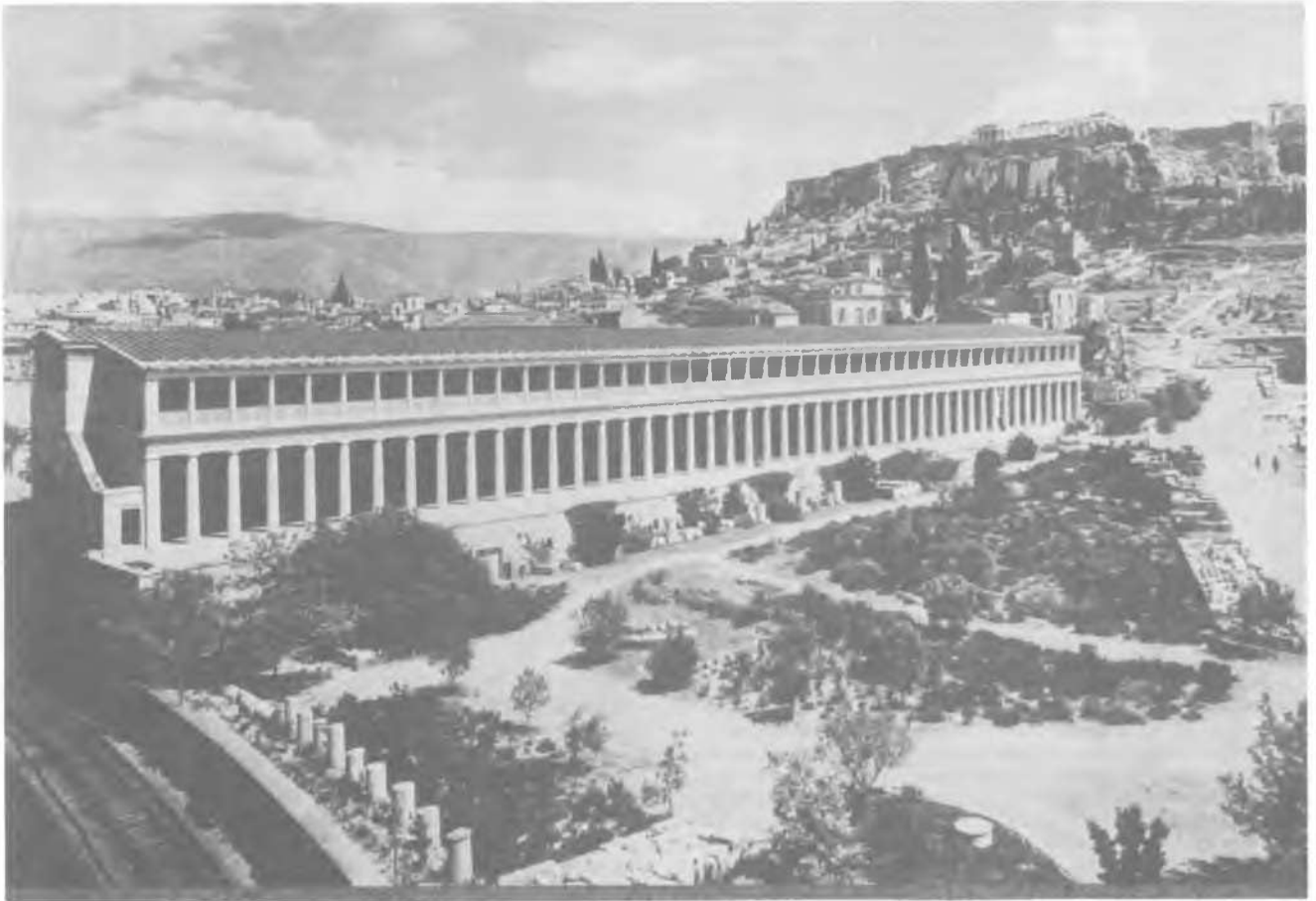
Fig. 27 - Reconstruction of the Attalus stoa in Athens (Perm. of the American School of Athens).
