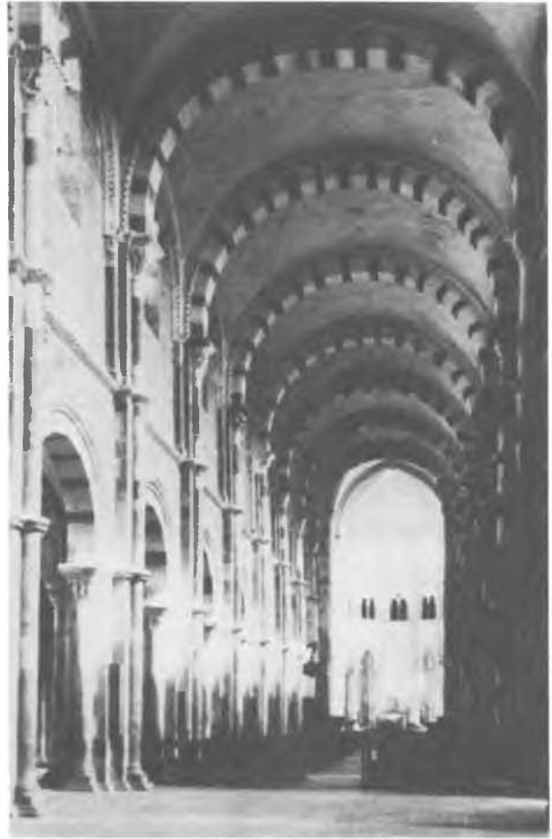
Fig. 46 - The basilica of Vezelay - Distortion of the vaults and pillars.
