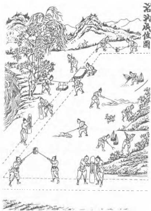
Fig. 31 - Sung Code of 1103. Site formation. The range of methods of compaction can be seen.
