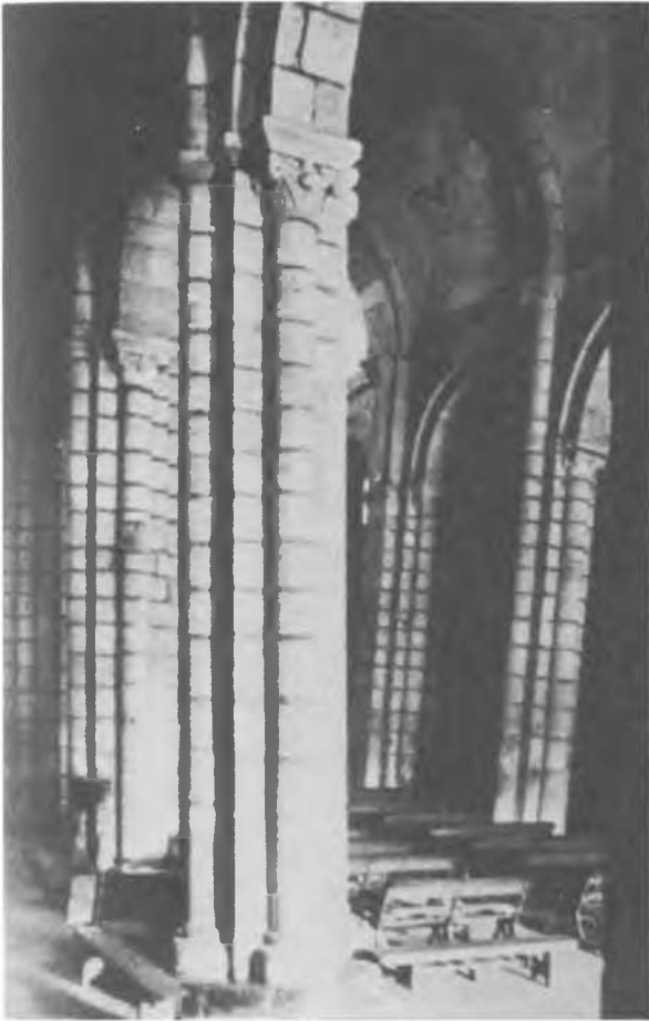
Fig. 45 - Santa Maria la Real del Sar - overturning.
