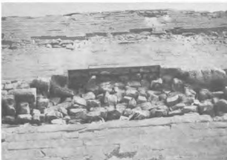
Fig. 59 - View of the filling material behind wall 6.
