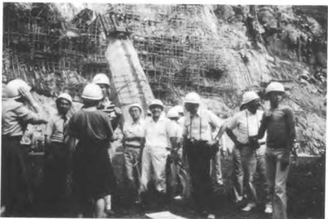
Tedorigawa Dam (Post Conference Tour)
