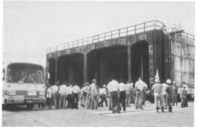
Submerged Tunnel (Technical Visit)
