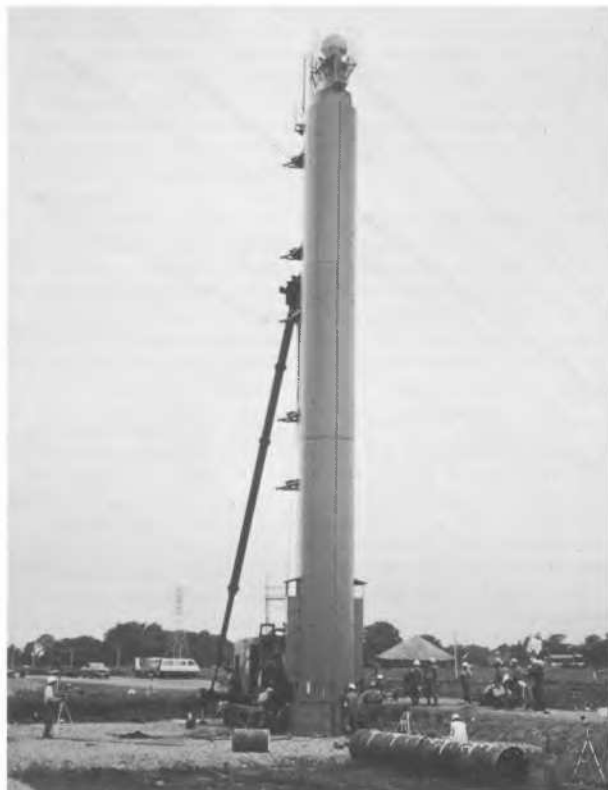
Driving a pile with the hood closed
