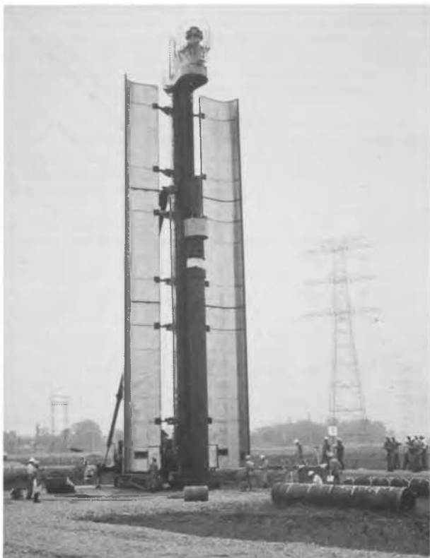
The hood opened before pile driving
