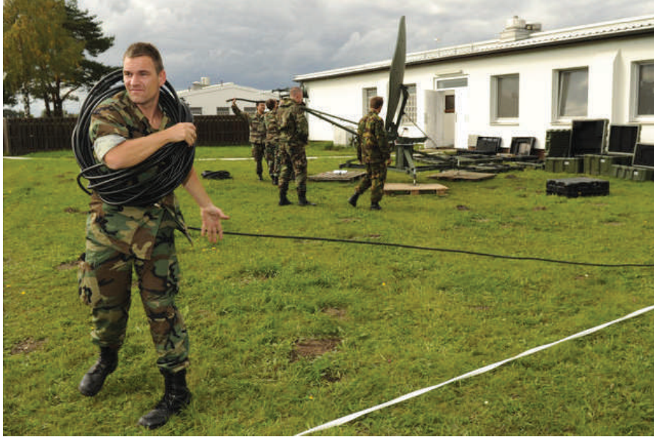
Photo 1. Combined Endeavor service members set up their work site in Grafenwöhr, Germany, September 16, 2010, during Combined Endeavor, a communications interoperability exercise that prepares international forces' command, control, communications, and computer systems for multinational operations. (U.S. Air Force photo by Staff Sgt. Tim Chacon/Released)
