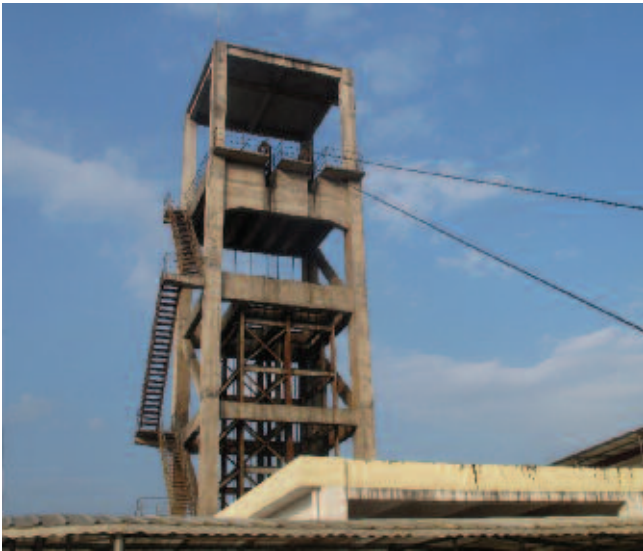
Figure 12: Head-frame: Maoping Mine, Jiangxi Province, China. Shaft access for personnel and material to the underground workings and transport of ore to surface by skip.
