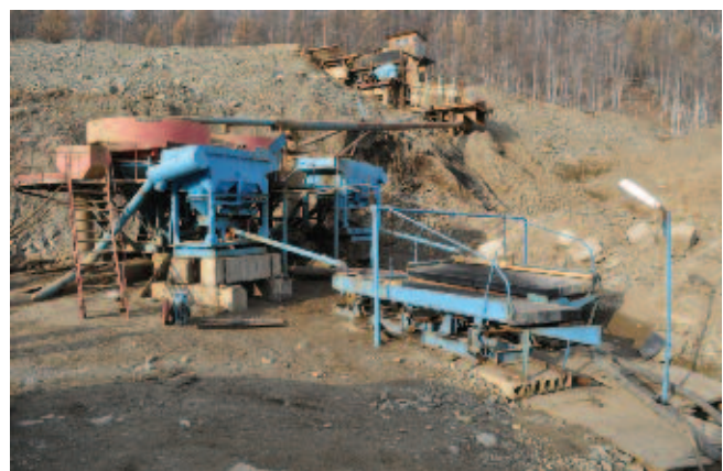
Figure 51: Alluvial mining : Compact modular gravity plant for seasonal operations in the Siberian summer at the alluvial wolframite deposit near Zakamensk, Burjatia, Russian Federation.
