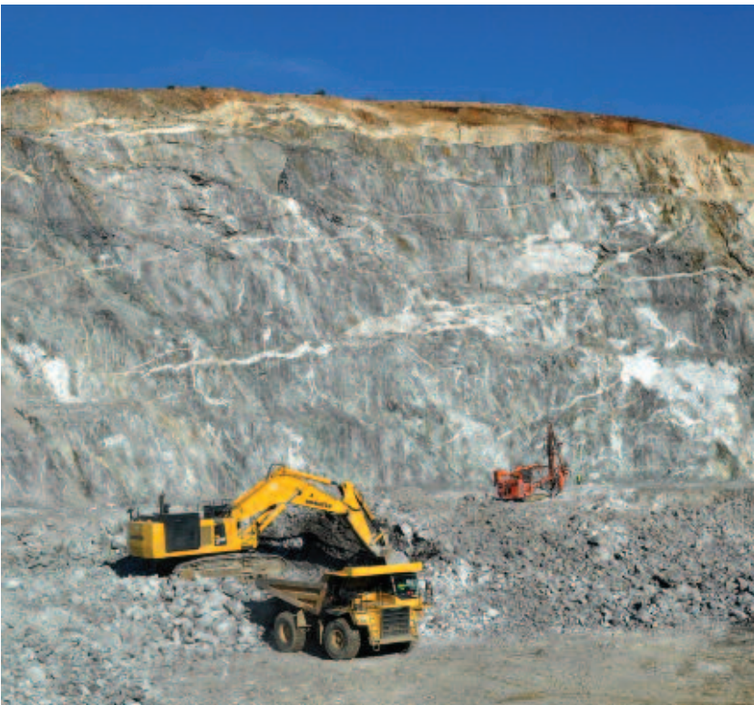
Figures 6 - 7: Open Pit Mining: Los Santos, Spain
