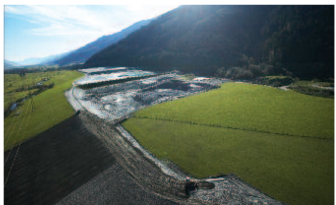
Figure 44: Continuous rehabilitation and re-vegetation of a tailings pond, Mittersill tungsten mine, Austria.
