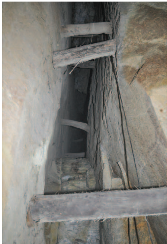
Figure 14: Narrow-vein open stoping, using timber props as support. Chollja, Bolivia. Vein zone is less than 1m wide.
