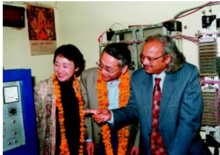
Yoshio Utsumi (in the centre), accompanied by his wife Masako, admires the 256-line capacity exchange at Runukat, which can work in rough environments without air-conditioning
