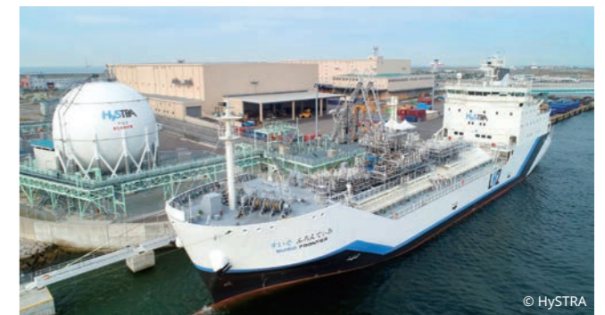
The Suiso Frontier, a liquefied hydrogen carrier
