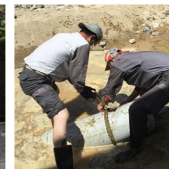
July 2018: Torrential downpours in western Japan
