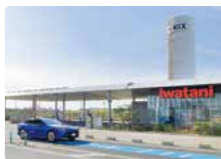
Iwatani Hydrogen Refueling Station at Kansai International Airport
