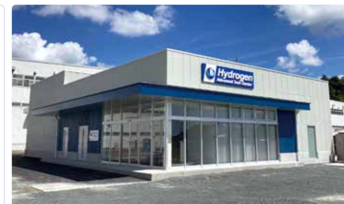
The Tokico System Solutions, Ltd. Hydrogen Advanced Tech Center
