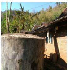
Figure 3. Rain water cistern
