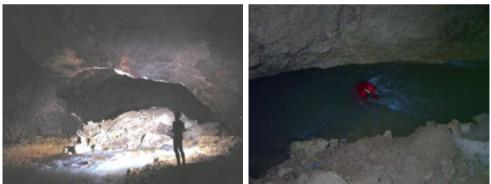
Fig. 9 Rock fall after downstream siphon (left) and open channel after blasting (right)
