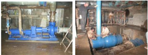
Fig. 11 First installed KSB-Module (left), Installation of VAG-valves at flood relief lines (right)
