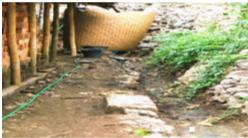
Figure8. Existing grey water discharge
