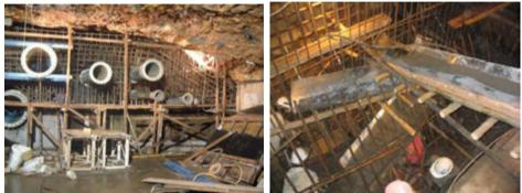
Fig. 10 Construction of the barrage with wall pipes (left), transportation of concrete in the cave (right)
