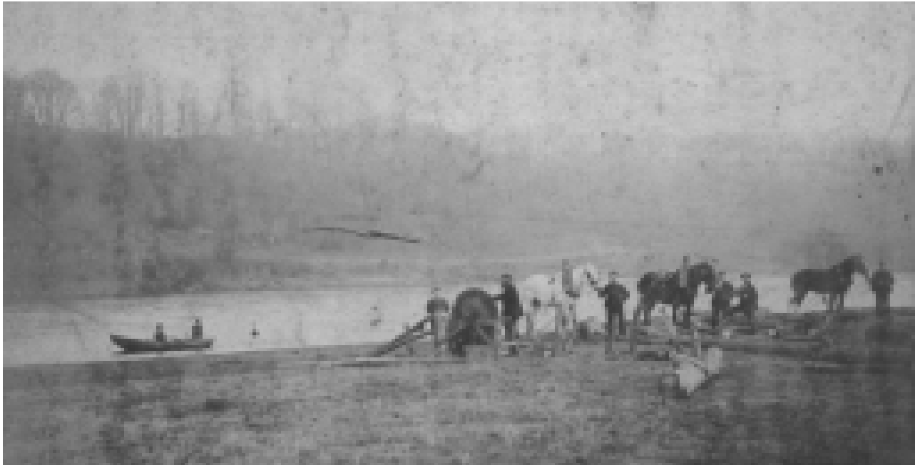
This early photograph is very faded but it shows timber being ferried across the river on a cable operated by the youngster and bearded man in the foreground. The three heavy horses will drag the logs from the riverbank to the sawmill.
