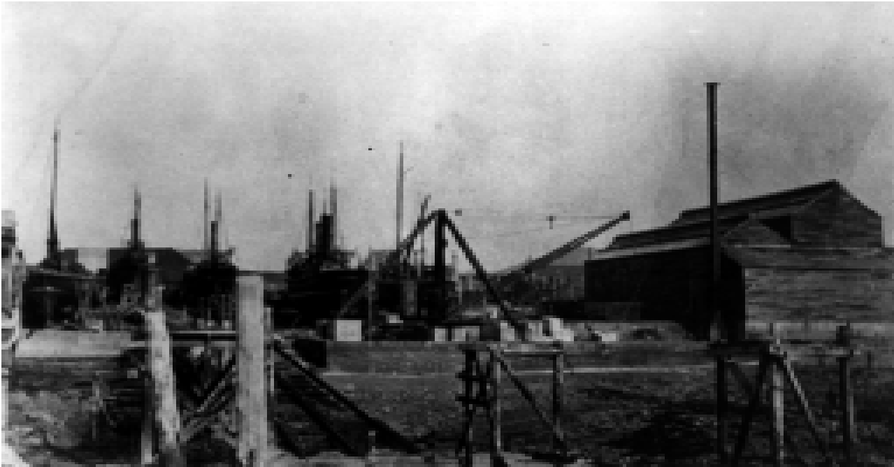
Steam drifters sit on the Jones Buckie slipway awaiting repair in 1925.
