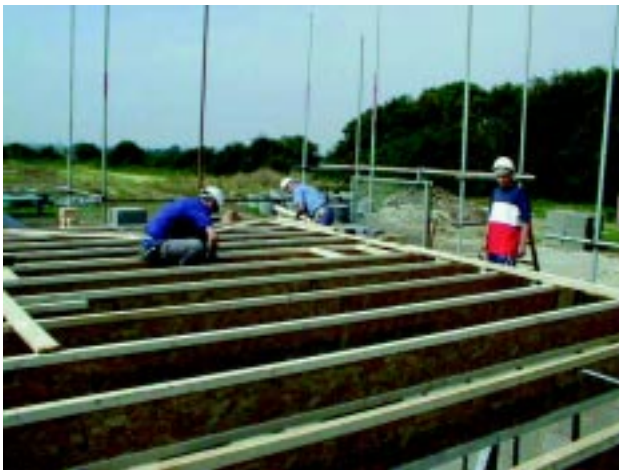
The I-Joists flooring system made by James Jones Timber Systems Division has been installed in houses all over the UK.
