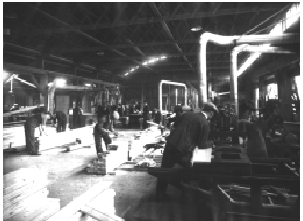
Two photographs showing work underway at the Larbert joinery works in the late 1920s. The man in the bowler hat in the centre of both pictures is the manager, Mr Steel.
