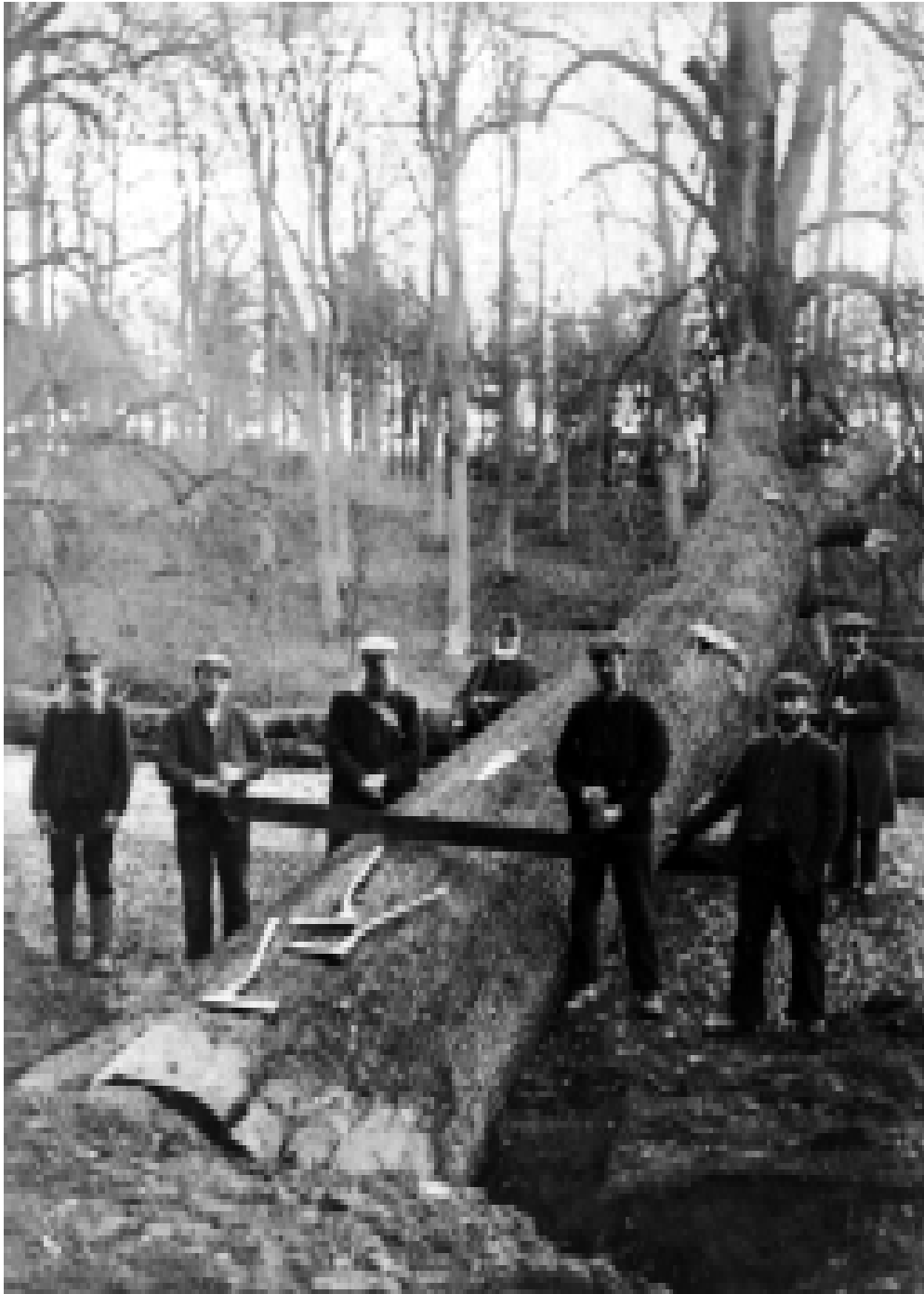
The photograph of this magnificent oak and the band of sawyers who felled it probably dates from around 1900. Note the four-man sawing team in the foreground. Two will pull on the saw itself while two heave on ropes attached to each end of the saw.
