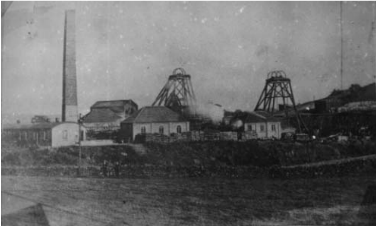
Collieries like this one, the Herbertshire colliery, near Denny, not far from Larbert, were common throughout Scotland at one time and represented one of the timber industry's biggest customers for several decades. Pit-props can be seen stacked up outside the colliery buildings. (Courtesy of Falkirk Museums.)
