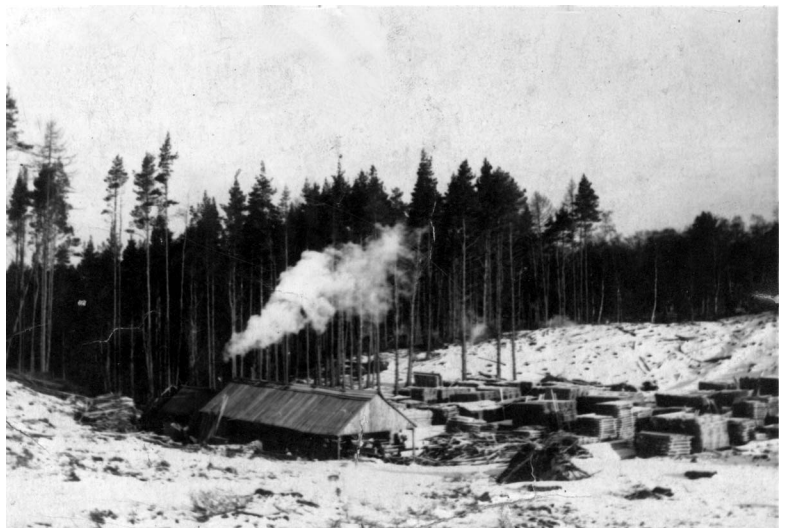
This wintry scene from the 1930s shows a typical forest sawmill located right next to the standing timber and surrounded by sawn timber. In the bitter cold, the steam engine is working hard.
