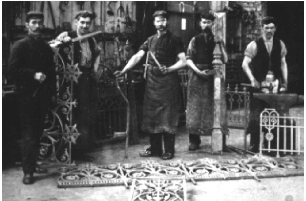
A group of Falkirk cast-iron foundry workers with the tools of their job and some typical examples of ornate cast-iron work. (Courtesy of Falkirk Museum.)
