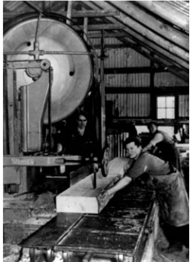
This is the interior of the new sawmill with a Stenner bandsaw installed at Castle Kennedy in 1951.
