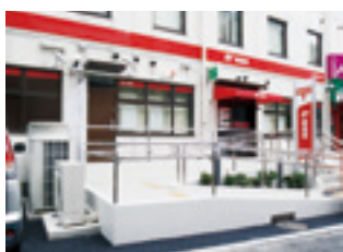
Ramp and handrails installed at the entrance
