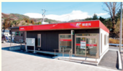
Sanriku Post Office following restoration (Iwate Prefecture)
