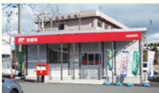
Temporary facilities for the Naraha Post Office (Fukushima Prefecture)
