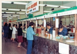
Paperwork at the postal savings counter/1983
