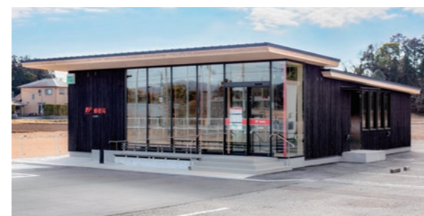
Maruyama Post Office (Minamiboso City, Chiba Prefecture)
