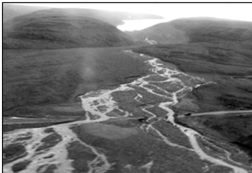
Figure 1. The road destroyed by the flood of an outlet stream of Qaanaaq Ice Cap. Photograph taken on 3 August, 2016.
