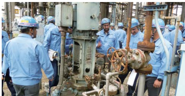
Problem-finding in a refinery (compressor)
