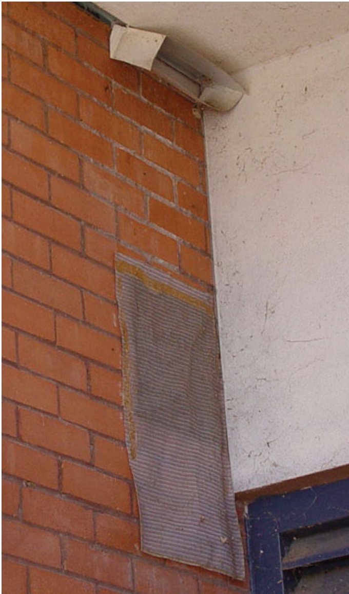
Figure 2. A temporary, one-way cover over holes allows bats to get out, but not back in.
