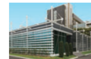
Customer Solution Lab (Chiba District)
