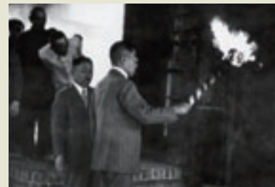
Blowing-in of first blast furnace
