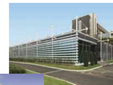
Customer Solution Lab (Chiba District)
