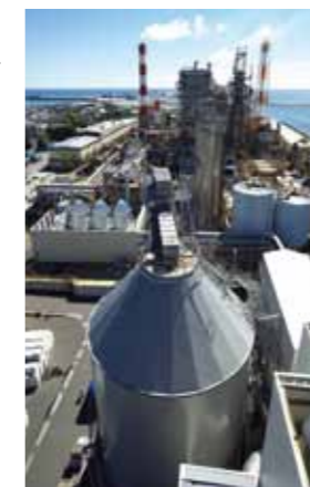
Wood biomass power plant
