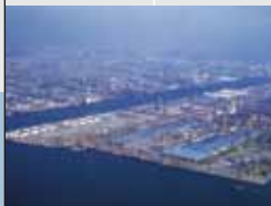
Completed Ohgishima (foreground)
