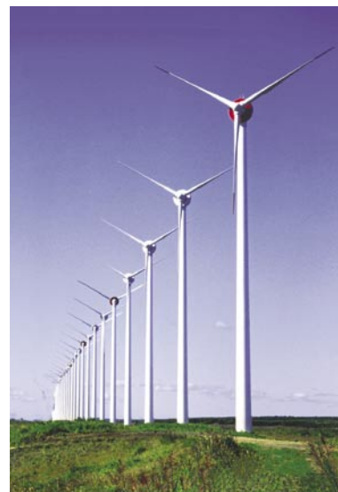
Wind power plant
