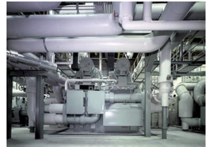
DHC system utilizing waste heat in sewage
