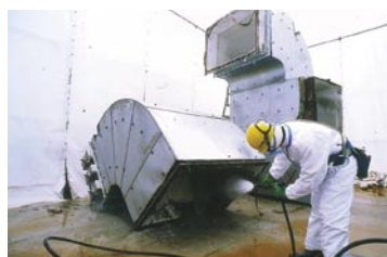
High-pressure water cleaning and removal of deposits
