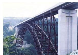
Oku-Aso Bridge constructed by using weathering steel
