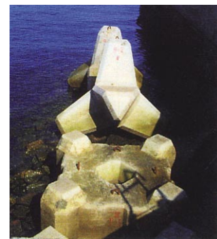
Wave-absorbing blocks made from steel making slag
