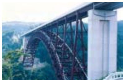
Oku-Aso Bridge constructed using weathering steel
