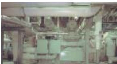
DHC system using waste heat in sewage
