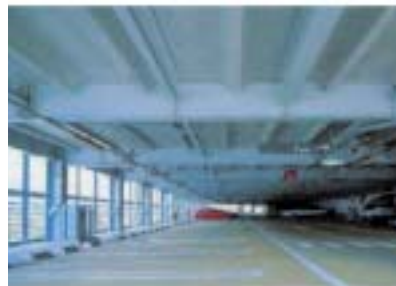
Parking building using fire resistant steel
