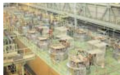
Polycrystalline silicon solidification plant
