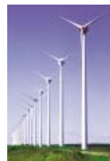
Wind power plant
