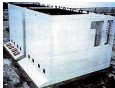
Seawater exchange-type hybrid caisson
