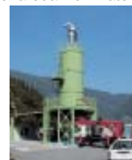
Driftwood recycling plant
