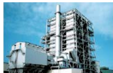
CFB boiler power plant
