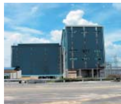
Papermaking sludge waste heat recovery plant
