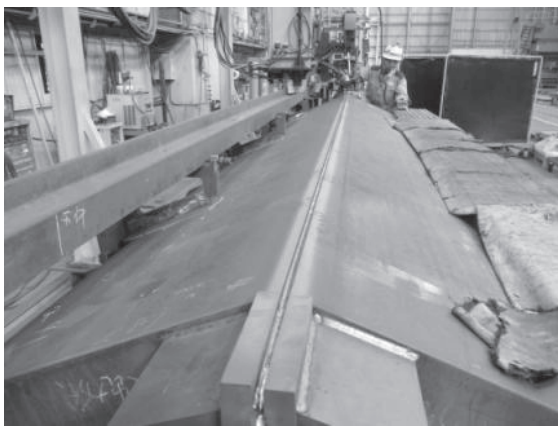
Photo 3 Adaptive control of the welding speed
