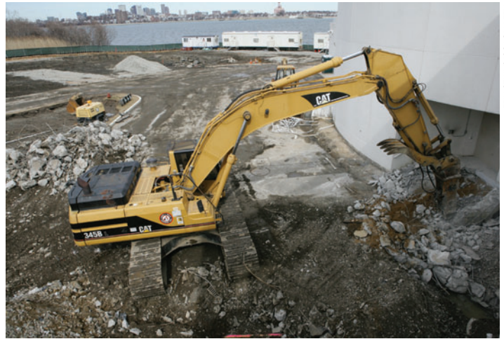
Construction begins on the shores of Dorchester Bay.
