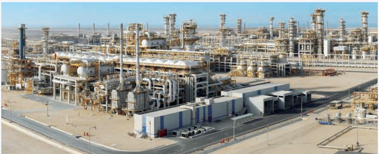
JGC constructed this large-scale gas processing plant in Qatar.
