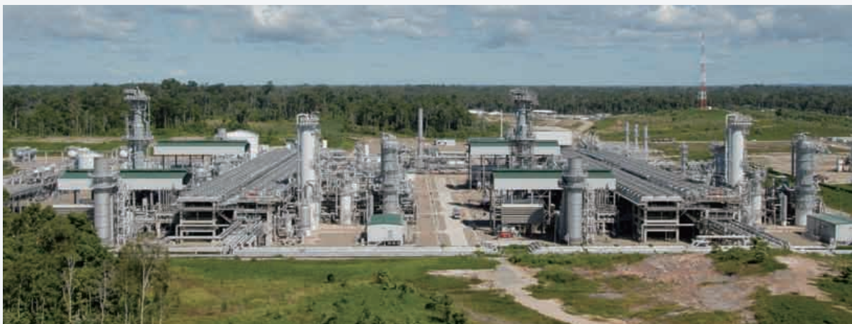
JGC constructed this large-scale LNG plant in Indonesia.
