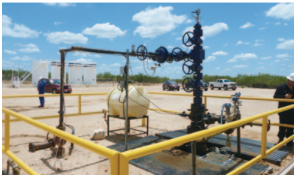
Completion rig (Eagle Ford)
