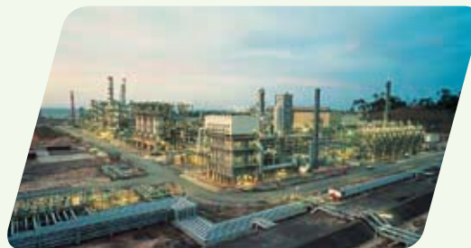
World's first commercial GTL plant, constructed by JGC, Malaysia
