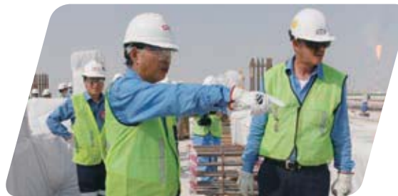
President Takeuchi patrols a construction site
