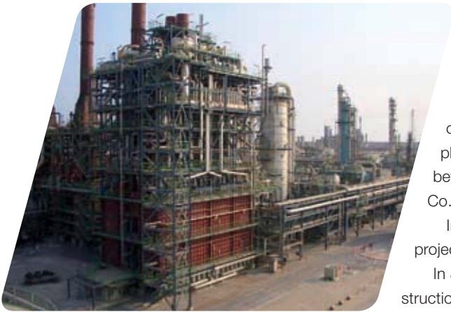
Ethylene facility expansion project for Qatar Petrochemical Company, Ltd., Qatar
