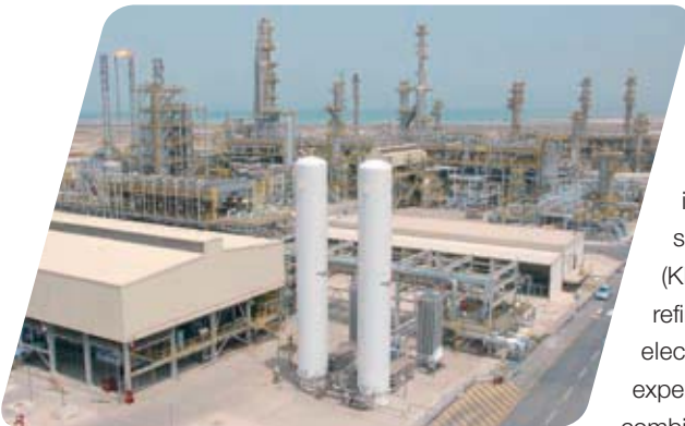
Petroleum refinery modernization project for BAPCO, Bahrain
