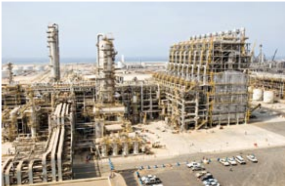
High olefin FCC facility and ethane crackers for Rabigh Refining and Petrochemical Company, Saudi Arabia
