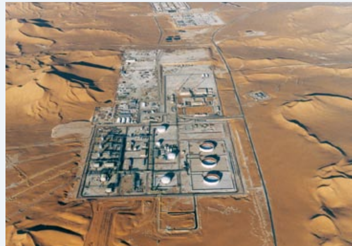
Crude oil recovery plant, Algeria
