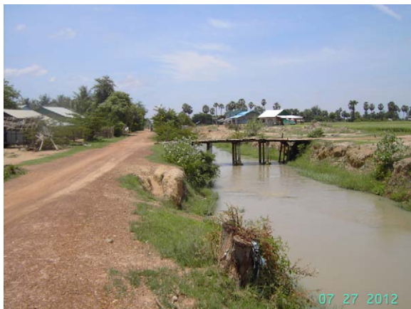
Existing south main canal
