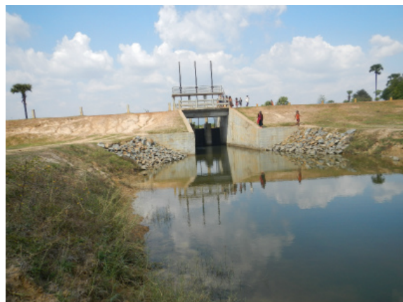
Intake of Khpob Krous Reservoir
