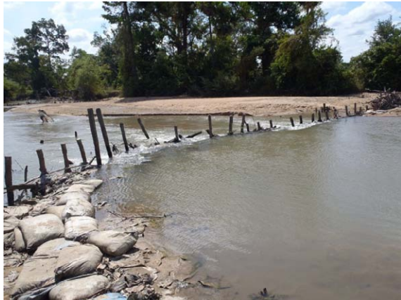
Temporary Weir for Daun Pue Intake made with Sand Bags and Wooden Material
