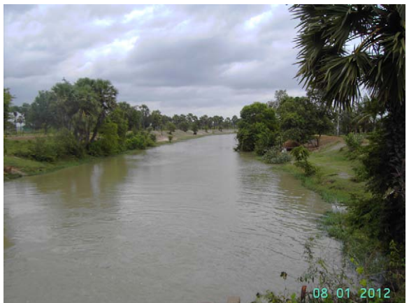
Existing north main canal
