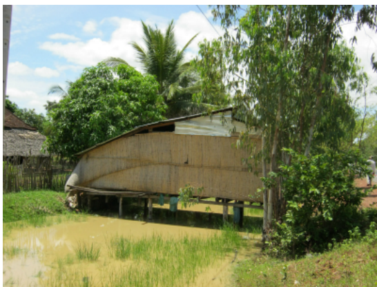
House on canal to be rehabilitated
