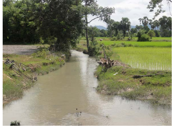
Main canal in Cheap Commune
