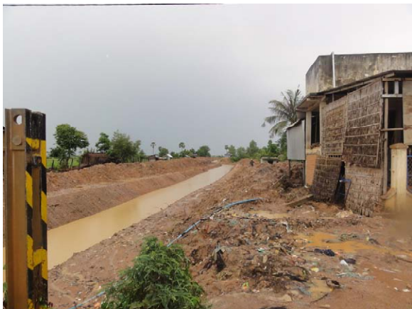
Rehabilitated Canal MR1 and illegal household
