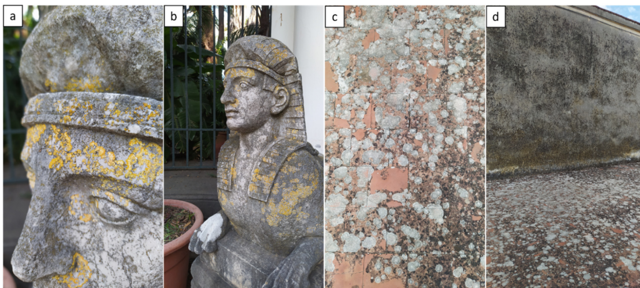
Figure 4. Lichens on statues representing sphinxes at the Botanical Garden of Portici (Naples, Italy) (a,b); and lichens on the roof of the Royal Palace of Portici (Naples, Italy) (c,d). Pictures by Alessia Cozzolino.
