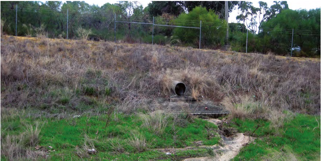
Figure 22: Fenced Off Sump at Lilburne Park
