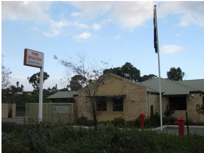
Figure 21: Duncraig Fire Station
