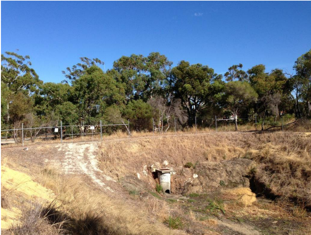
Figure 31: Fenced off Sump at Warwick Open Space
